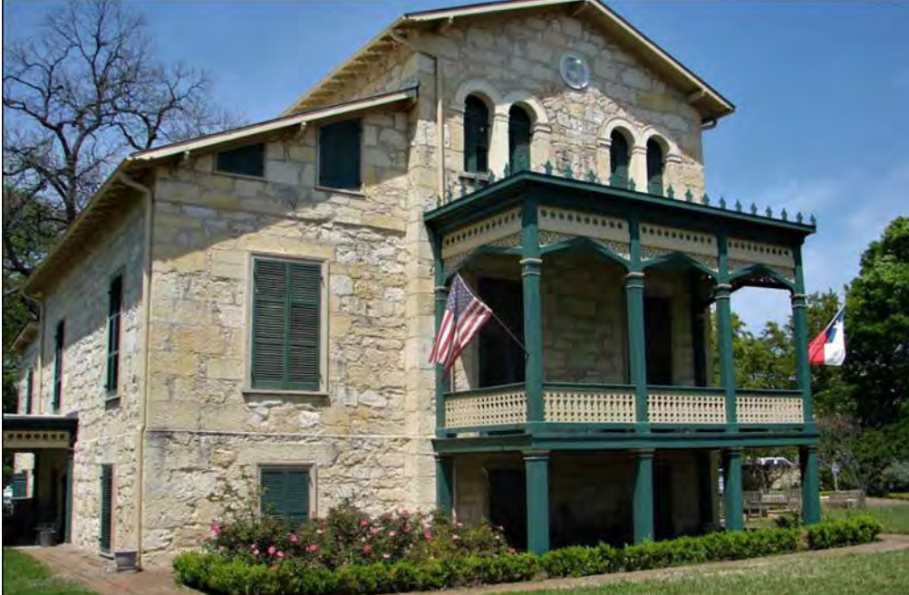
FIGURE 2-7. Headquarters of the San Antonio Conservation Society are located in the Anton Wulff House in the King William District. The home was built between 1869 to 1870 by German immigrant Anton Wulff, who became the city's first park commissioner. The organization saved the house from demolition and restored it in 1974. Source: San Antonio Conservation Society
