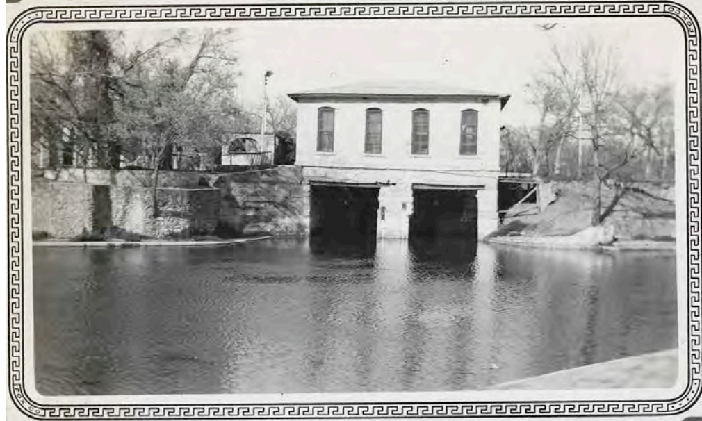
FIGURE 10-6. Circa 1940-1950s photograph of Pump House No. 1, perhaps the oldest intact industrial building in Brackenridge Park, constructed in 1878 and located on the San Antonio River in Brackenridge Park. Source: Witte Museum Collection
