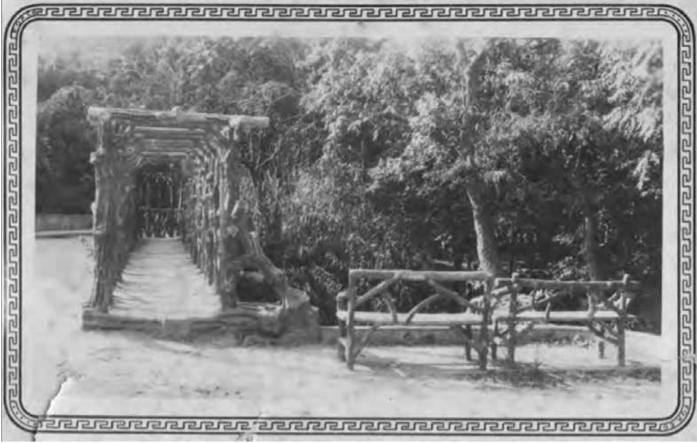
FIGURE 11-33. The Rodriguez Wooden Footbridge has 33 pairs of vertical tree trunks and resembles an arbor. Source: University of Texas San Antonio.
