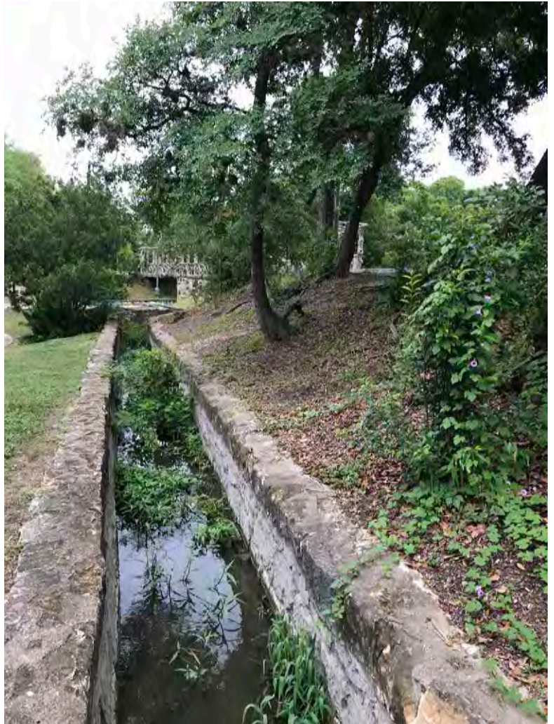
FIGURE 13-39. View of the historic irrigation channel that delivered water to Pump House #1. Source: Suzanne Turner Associates.
