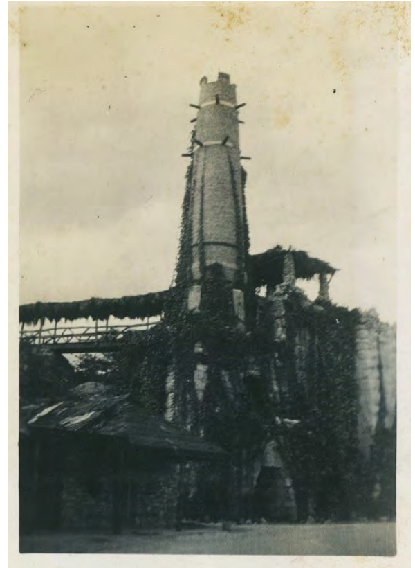
FIGURE 10-8. The Portland Alamo Cement smokestack, circa 1920s. Portions of the Japanese Tea Garden structure are visible behind the smokestack. Source: Witte Museum Collection, Image #1986-117G(5)
