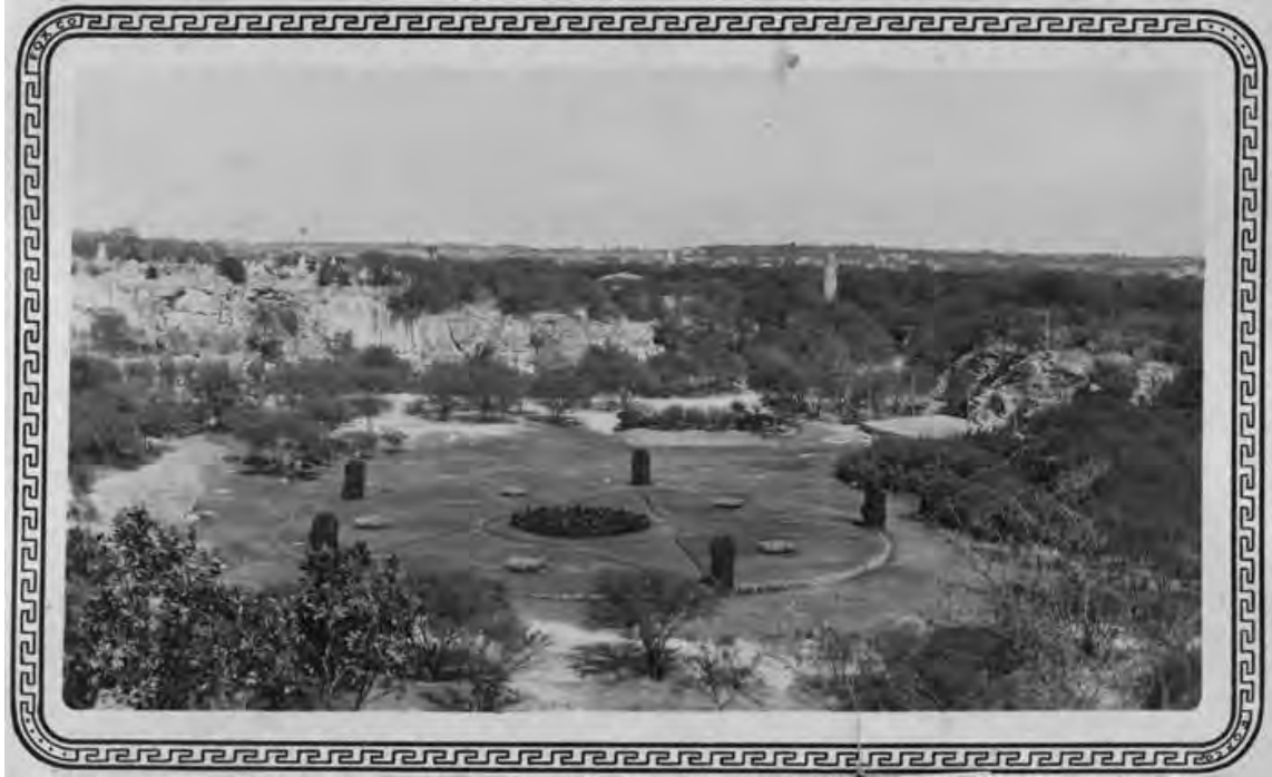
FIGURE 11-25. In the far right side of the postcard, you can see the original stage that was used for outdoor choral and theatrical performances. Later, the state became the site of the Sunken Garden Theater, which was enlarged and expanded during preparations for the Texas Centennial of 1937. Source: Witte Museum Collection
