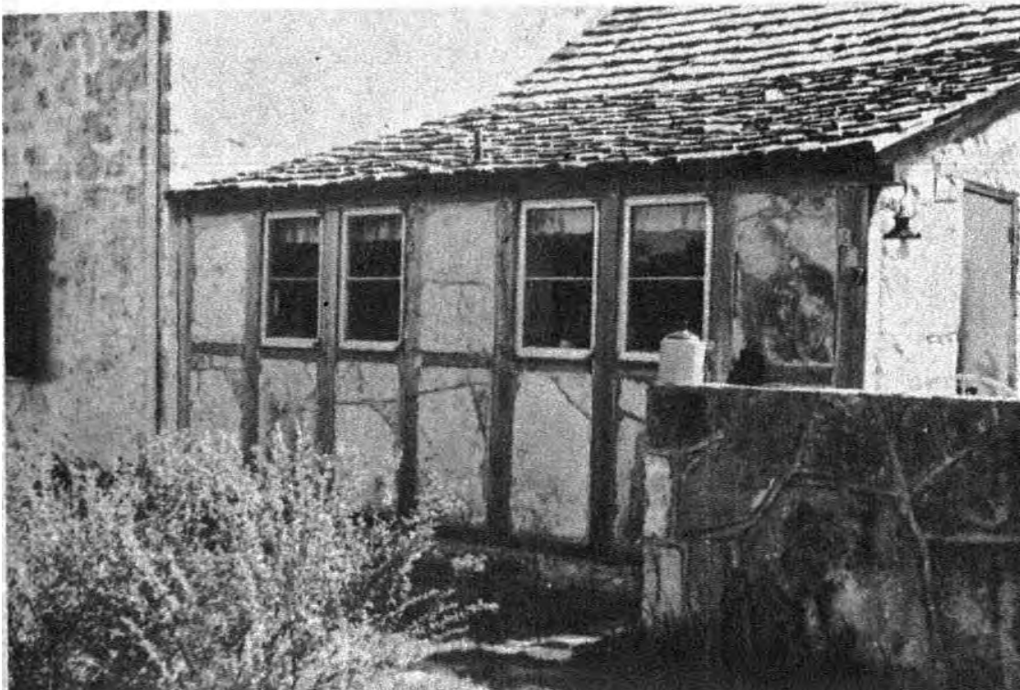
FIGURE 5–8. Two circa 1857 half-timbered houses in Kendall County, located northwest of Bexar County. The traditional German building method in which squared-off jointed timbers are secured with wooden pegs, and sometimes left exposed on the exterior of the building. These homes illustrate the method in combination with native Texas limestone. Source: Jordan-Bychkov, German Seed in Texas Soil , Figure 5.
