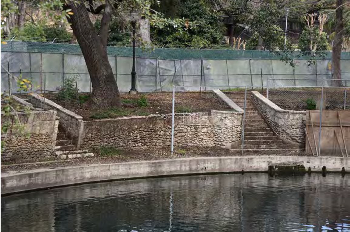
FIGURE 13–11. View of river walls, southwest of bathhouse, February 2019. Source: Reed Hilderbrand
