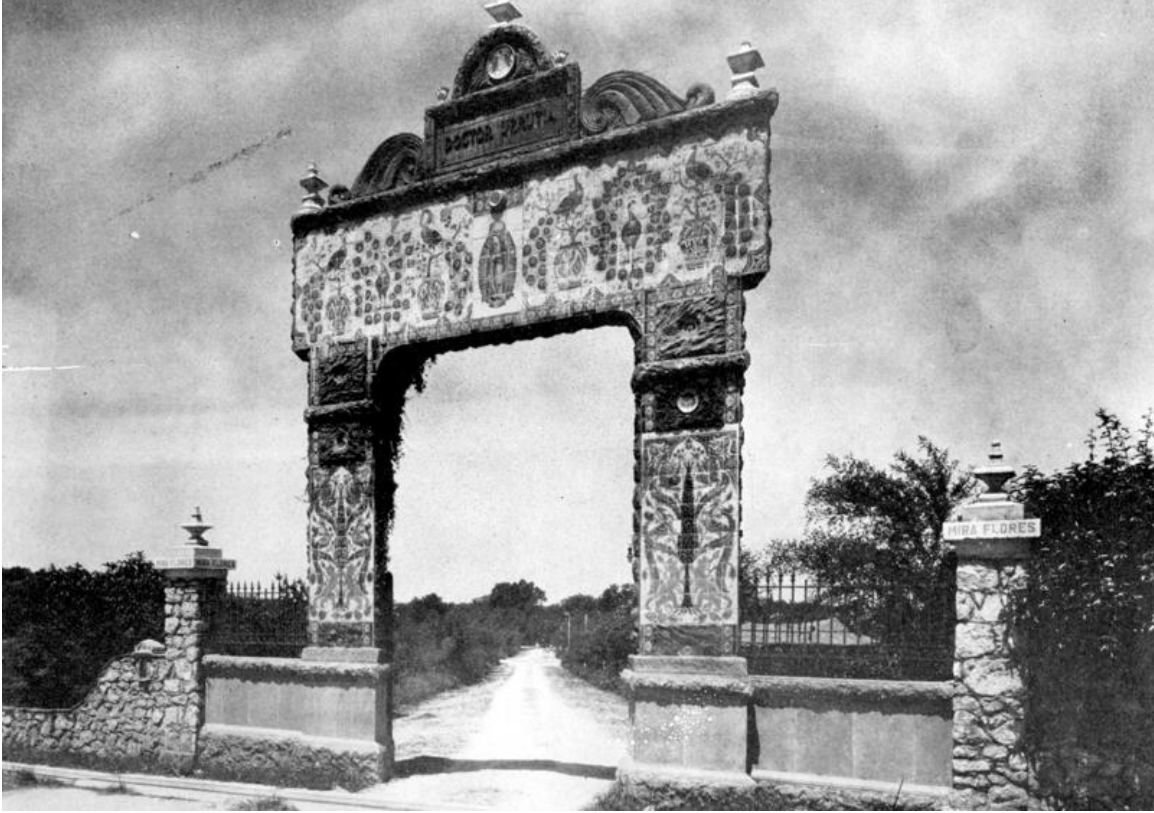
FIGURE 11-28. Miraflores arch of Spanish Talavera mosaic tile. The structure originally stood near the corner of Broadway and Hildebrand Avenue and is now at the San Antonio Museum of Art. Source: Texas Public Radio, www.tpr.org/post/mystery-behind-san-antonios-miraflores-park-uncovered
