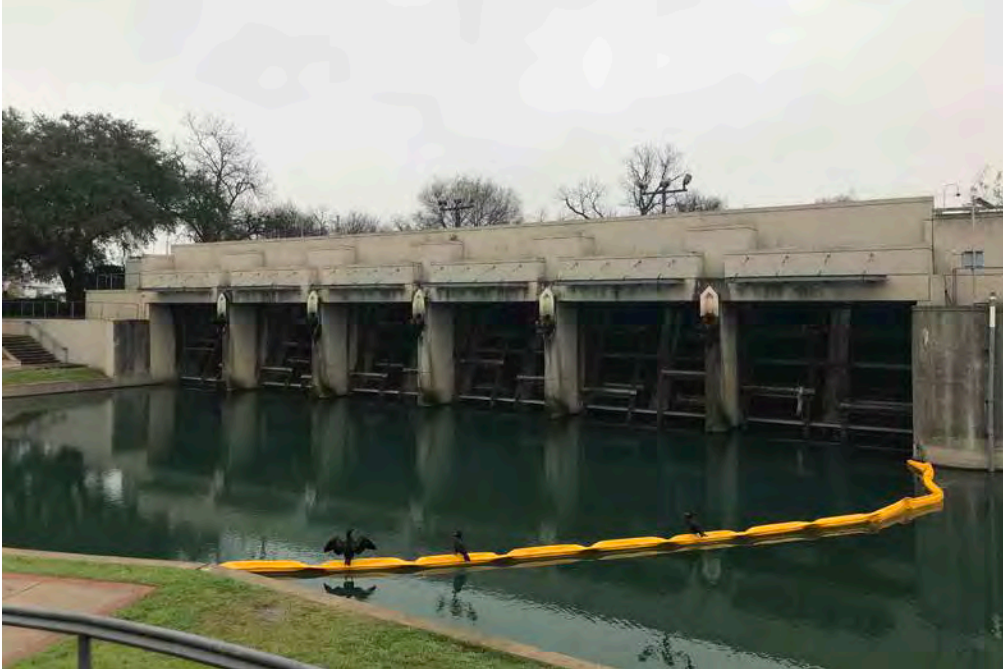
FIGURE 1–8. Photo of Inlet Tunnel flood control structure at Josephine Street. The structure became operational in 1997 and prevented a major flood the following year. Source: Reed Hilderbrand
