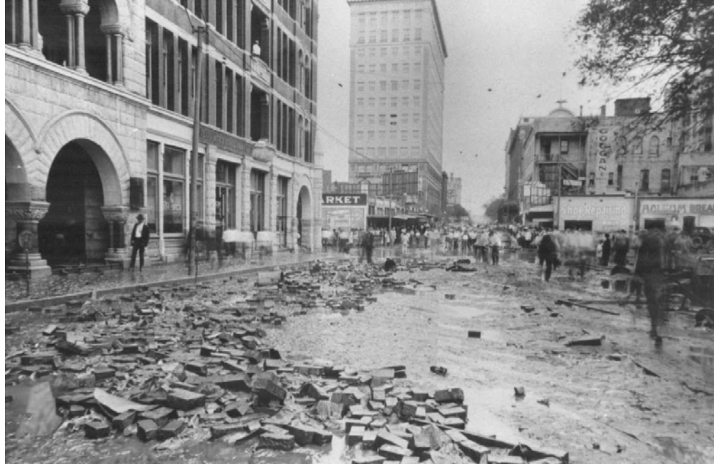
FIGURE 2-8. Navarro Street after 1921 flood, the worst flood on record in San Antonio in terms of loss of life and property. Note the mesquite block paving floating. Source: San Antonio Express-News Archives.
