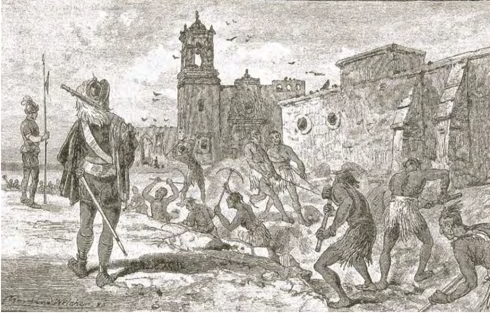
FIGURE 9–2. Engraving of Indigenous people building the acequia at Mission San José between 1720–1730. Source: Weckler, 1883, published in Charles R. Porter, Jr., Spanish Water, Anglo Water
