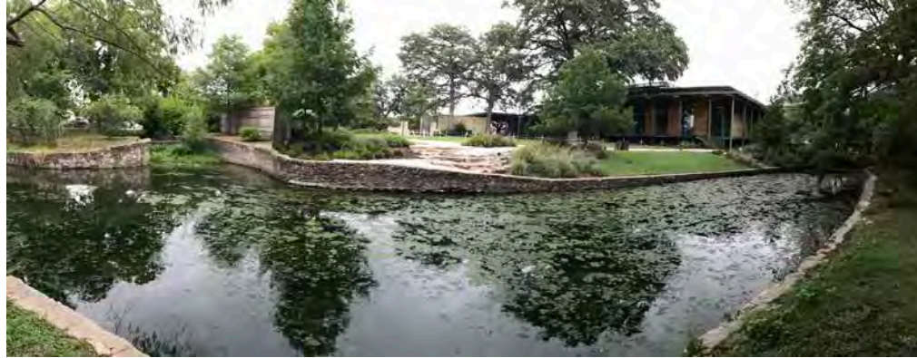
FIGURE 13–44. View of the back of the Witte Museum, looking across the San Antonio River. Source: Reed Hilderbrand
