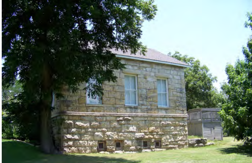
FIGURE 13–28. View of stone architecture, lower pumphouse number two. Source: Reed Hilderbrand
