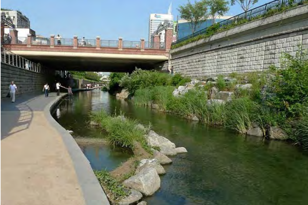
FIGURE 1–3. View of the Cheonggyecheon Stream after removal of the elevated highway. Areas were built into the stream to slow water and support bird and aquatic biodiversity. Source: Alexander Robinson, published in “Cheonggyecheon Stream Restoration Project”
