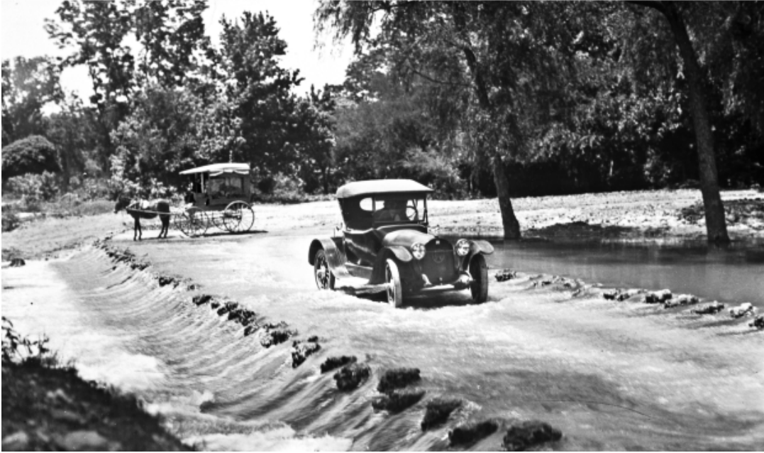
FIGURE 11-20. An automobile drives through the low-water crossing at Tuleta Drive. Juxtaposed in the background is a small horse and carriage. The early configuration of the crossing shows random-sized stone as edge markers. Later, the stone was replaced with elevated concrete “pads” to allow pedestrians to cross in a safer manner. Source: Jay Loudon, Work5hop.
