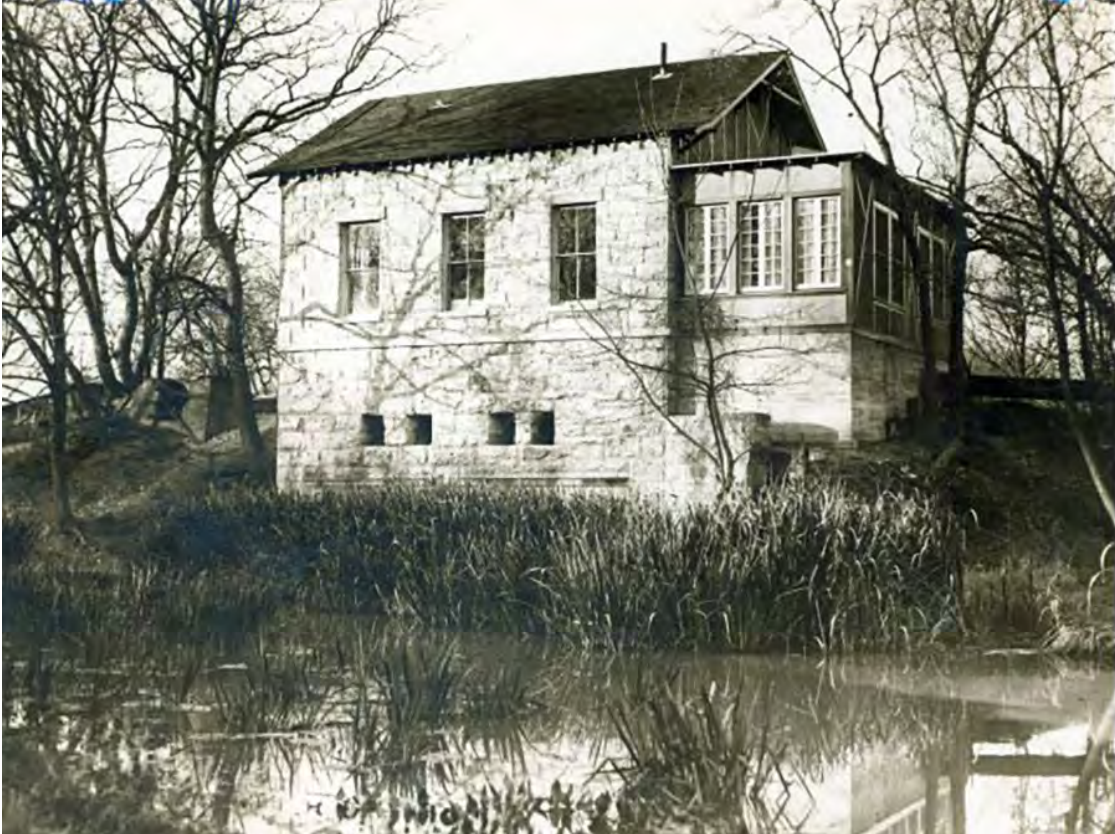
FIGURE 5–9. The lower pump house in Brackenridge Park, constructed in 1885. German half-timbering construction melded with native limestone material can be observed in other places in the park, including the Japanese Tea Garden, where Mexican building methods are also seen, and the amalgamation of cultures is more pronounced. Source: Brackenridge Park Conservancy
