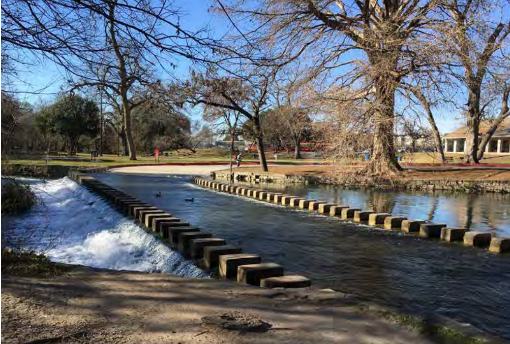
FIGURE 13–50. View of low-water crossing on Tuleta Drive. The Eleanor Brackenridge Playground and Brackenridge Park Conservancy office are visible in the background. Source: Reed Hilderbrand
